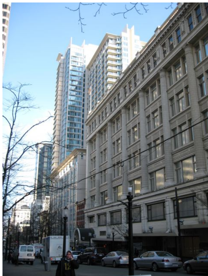
The Hudson on Granville at Dunsmuir is an example of residential development in the heart of Vancouver's business district.
